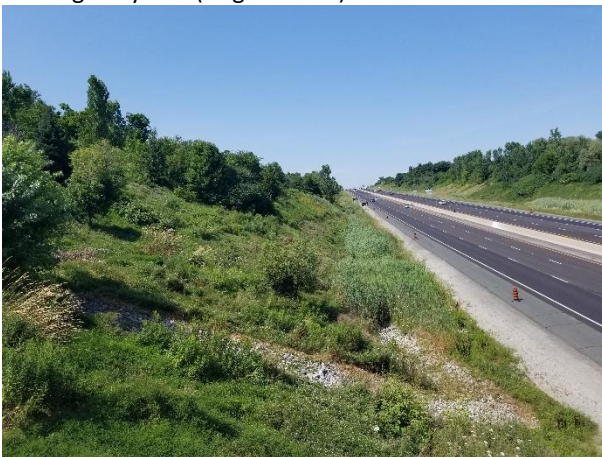
Plate 19: Embankments adjacent to Highway 407 at Upper Middle Road overpass (August 2019).
