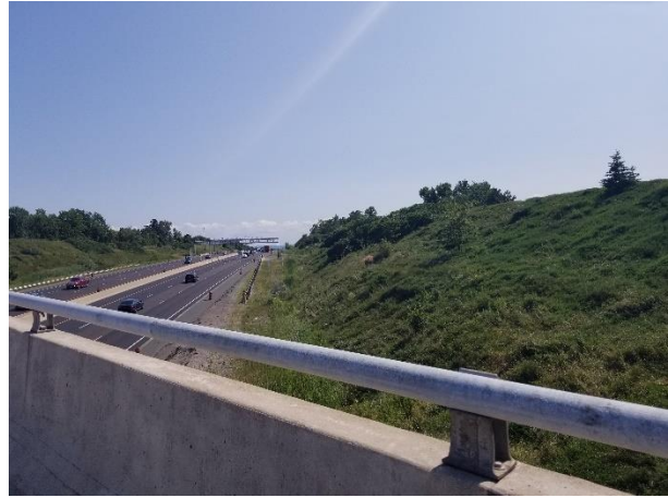
Plate 18: View of the embankments next to Highway 407, looking south from the overpass at Guelph Line (August 2019).
