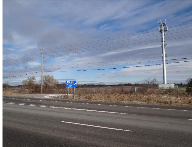
Plate 14: Proposed station location at Bronte Road at Highway 407, looking northeast (November 2018).
