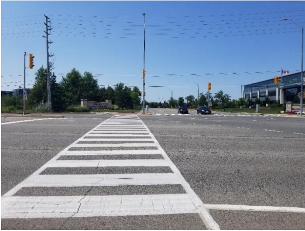
Plate 5: Intersection of Mississauga Road and Hereford Street, looking northwest (August 2019).
